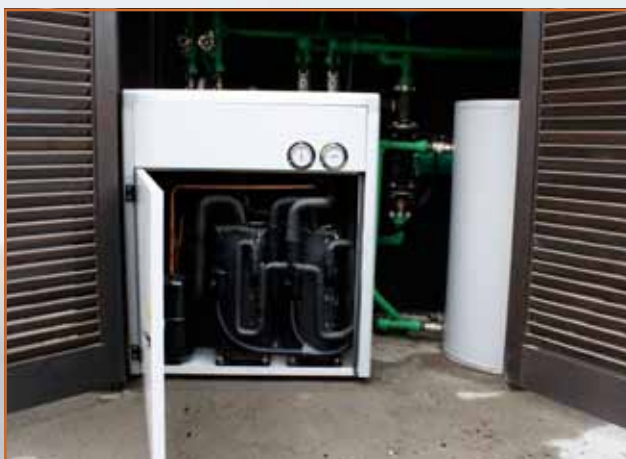
The heat pump unit is mounted discretely in an outdoor locker.
