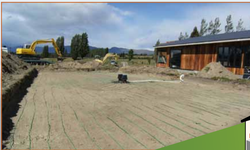
The "captor field" being installed.
