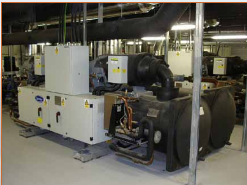
Chillers used to heat and cool the water for use throughout the airport.
