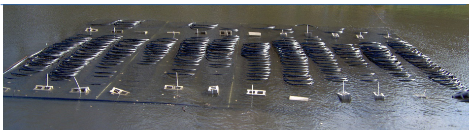
Figure 20. Submerged loop ready for sinking and anchoring
