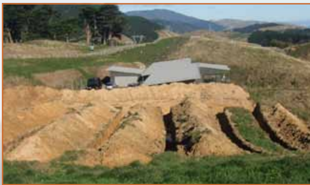
The slinky coils are installed in a network of trenches.
