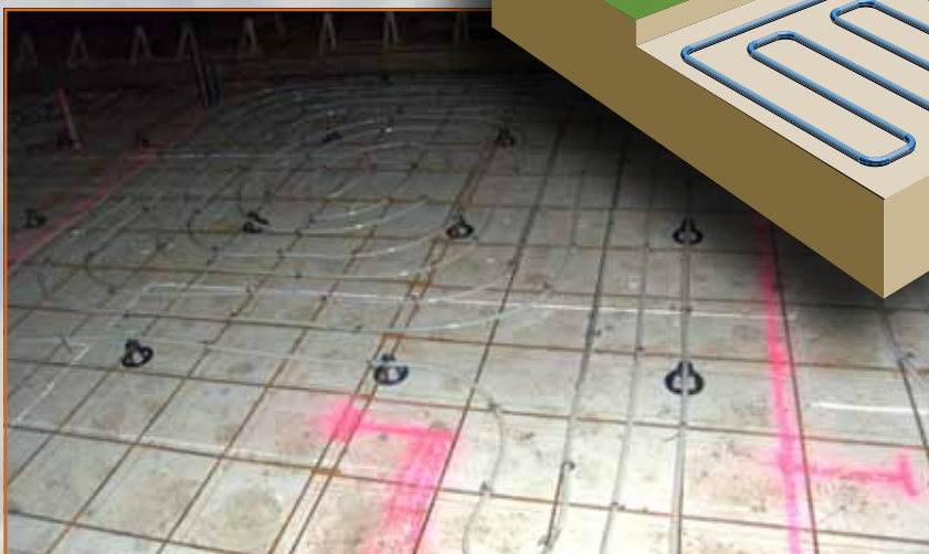
The under floor heating system. Heat generated by the captor field is used to heat water that is circulated through these pipes, installed in the concrete slab foundation.
