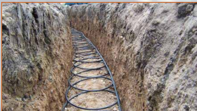
The 'slinky' pipes laid in the trench.
