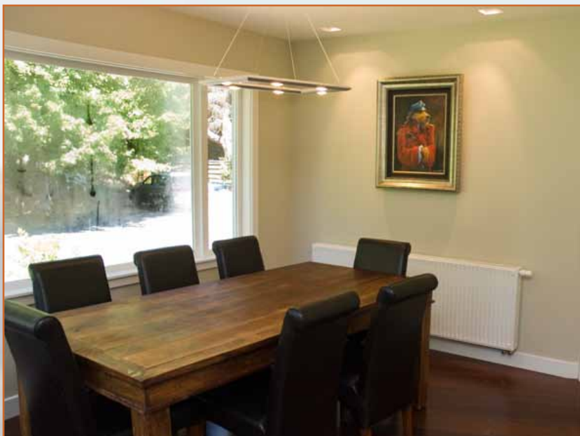
Warm water generated by the heat pump is circulated through radiators.
